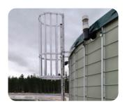
**Platforms** Steel or aluminium platforms and ladders, as well as wrap around staircases and walkways.
