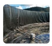
KlipJet By introducing oxygen into the system, KlipJets promote ongoing aerobic biodigestion of the wastewater, accelerating its decomposition and reducing odours.
